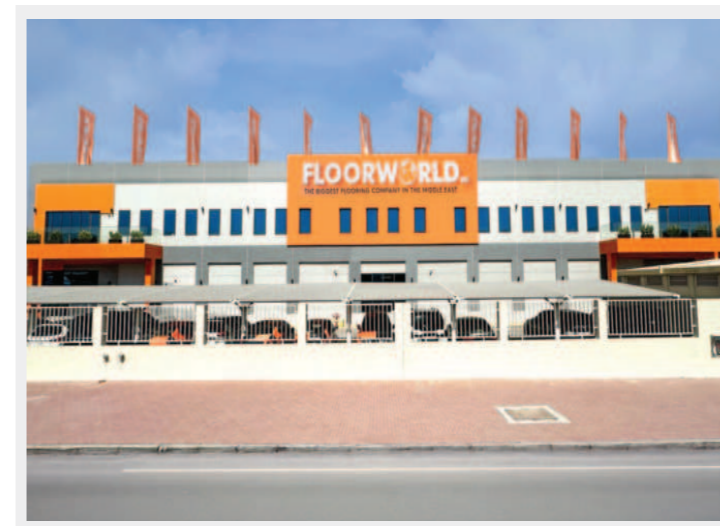
Regional Headquarters Dubai Investment Park-2, Dubai, UAE
